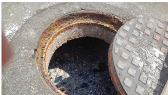
Fig. 6 Anaerobic reactor as seen through manhole
